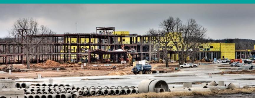
The last of 442 concrete underground piers were installed in July 2008. A massive 2,800 tons of steel have been erected at the site. In addition, 750,000 square feet of concrete paving is near completion. Roofing on the hospital, clinic and central plant is complete. Interior wall framing
