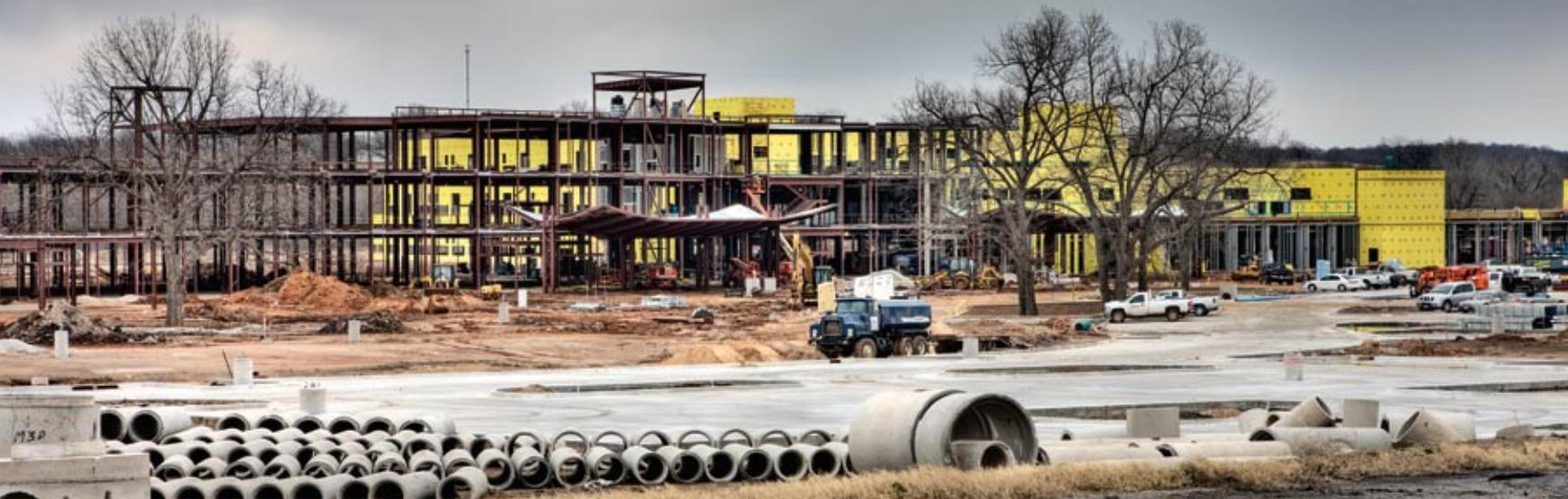
The last of 442 concrete underground piers were installed in July 2008. A massive 2,800 tons of steel have been erected at the site. In addition, 750,000 square feet of concrete paving is near completion. Roofing on the hospital, clinic and central plant is complete. Interior wall framing
